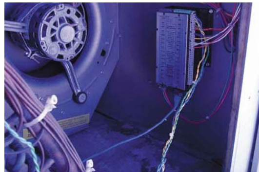
Poorly tuned commercial heating-ventilation-air conditioning systems can easily lose 25-30% of their effectiveness. One solution is the Rooftop Diagnostician, a PNNL innovation shown on the right. This electronic intelligence unit sends detailed information on operating status and provides remote tuning capabilities. Within homes, offices, stores and factories, internal networks of sensors and microprocessors will produce tremendous energy efficiency gains that could shave $15 billion off power bills through 2020.
