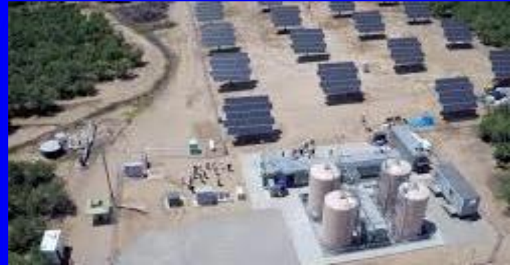
Enervault 250 kW 4-hr Irpn-Chrome Flow battery. Turlock Ca.
